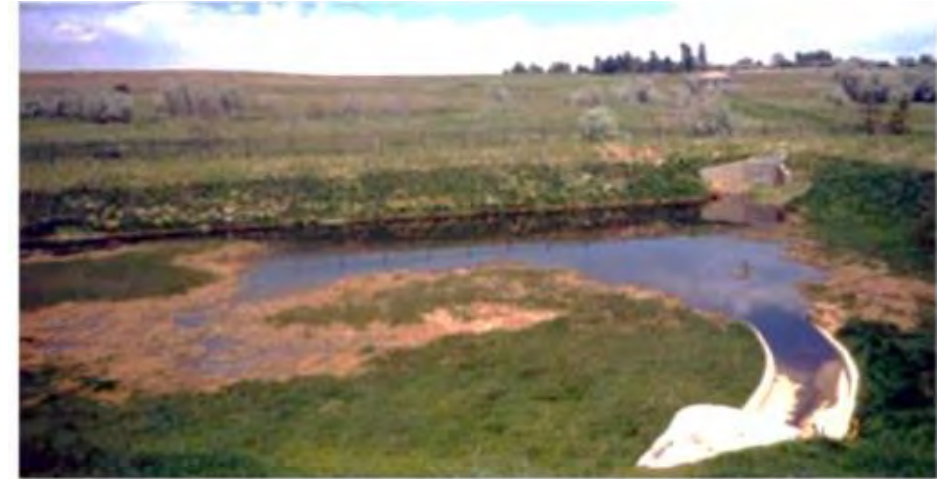
Extended Detention Basins
