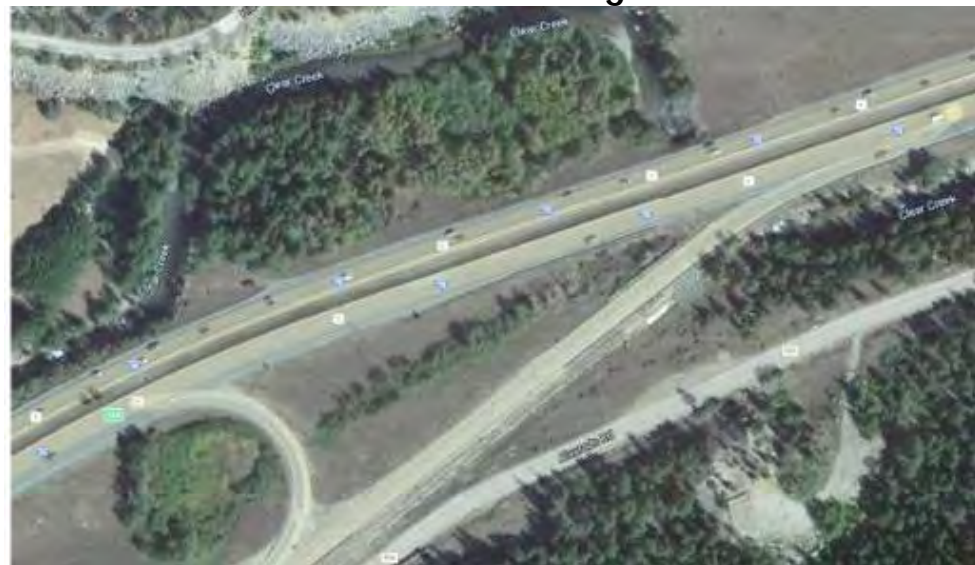
Constructed Wetlands and Engineered Ditches
